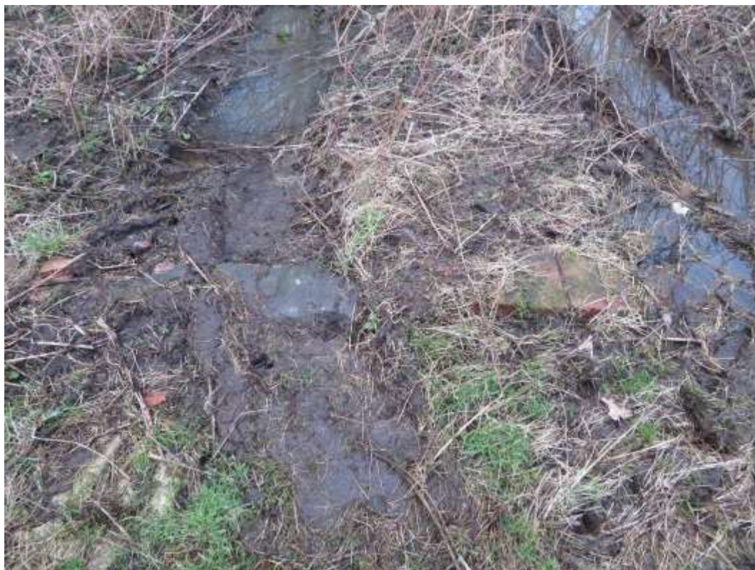
Plate 6 The foundations of a brick building can clearly be seen, as well as recent vehicle tracks across the moated platform
